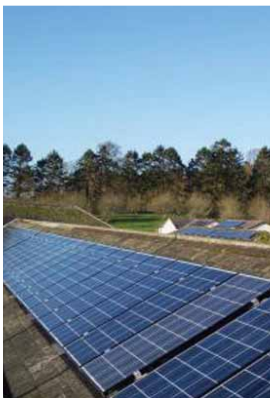
Bronllys Hospital, Powys is the first UK NHS hospital to generate electricity from sunlight. A 60.62 kW photovoltaic array reduces the hospital's need for fossil fuels.
